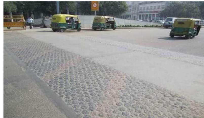
Photo 5.3 Tabletop with cobble stone on slope and cement concrete surface on top
